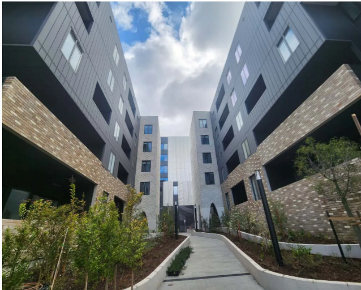
ኣብ Abbotsford St North Melbourne ዝተሃንጹ ሓደስቲ ሓይሊ ዝቐጥቡ ገዛውቲ ኣብ 2025 ተኸፊቶም እዮም።
