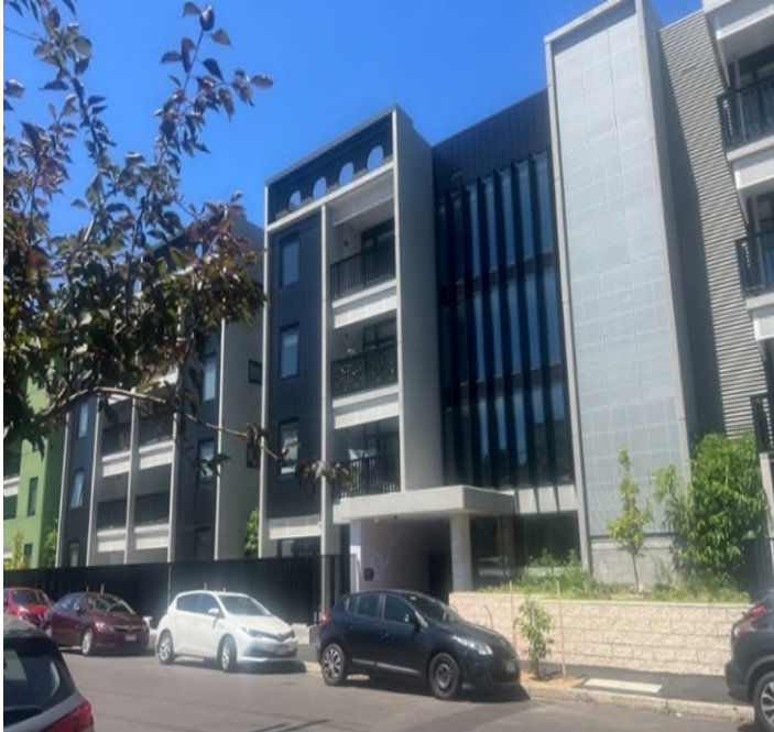
New, energy-efficient homes built on Victoria Street, Flemington, opened in 2024.
